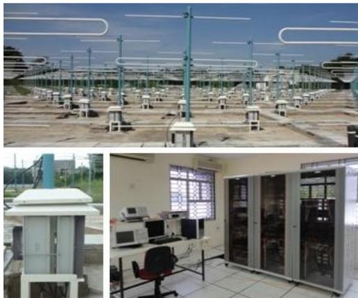
Fig 3: Photographs of pilot active array at NARL (a) Array field (b) TR module (c) Control and instrumentation room
