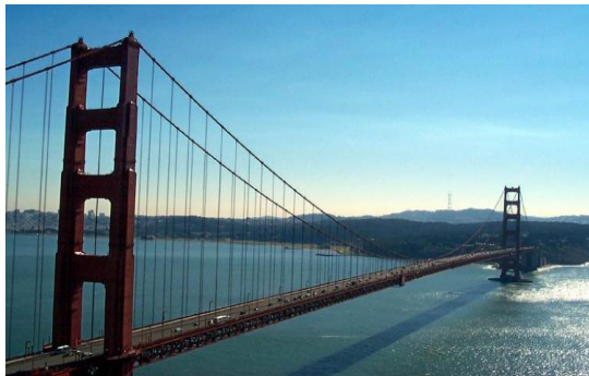
Fig 2: Implementation of SHM on Golden Gate Bridge
