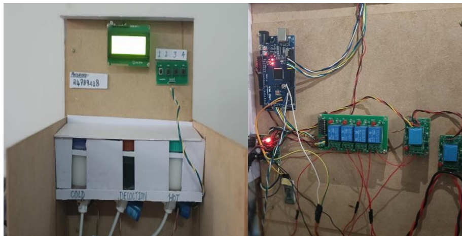
Fig 6: Motor Pump and Relay
