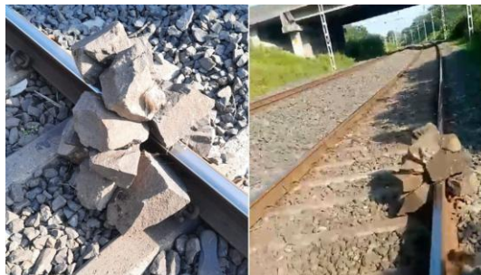
Figure 2.2 Stones on track
